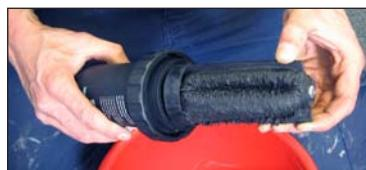
**CLEANING AND SERVICING** For optimum efficiency, clean out annually. Have a 750ml (min) container ready. Isolate heating system and close both valves. Open air vent (5). Using the spanner included in the pack open the drain valve. Drain all contents and then firmly close the
